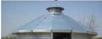
The louvered outer roof provides constant shade for the primary roof decking, creating a barrier to prevent overheating of the interior of the unit. Louvers in the outer roof allow the hot air to escape, while allowing rain water in for collection at the eave.
